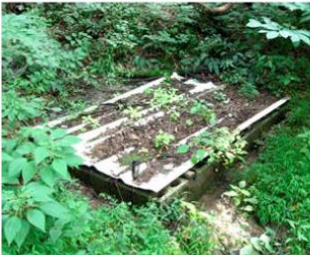
Photograph 7. The spring-fed cistern below the well pad. The cement block cistern is covered with sheets of metal roofing and its overflow drainage is visible in the foreground.
