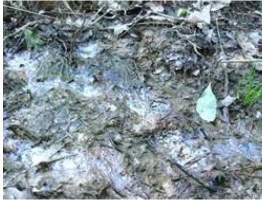
Photo 1. Oil sheen on mud in ditch behind tank.
