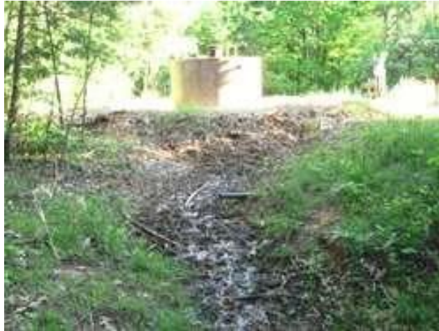
Photo 5. Ditch behind and below tank. The ditch goes a short way down hillside.
