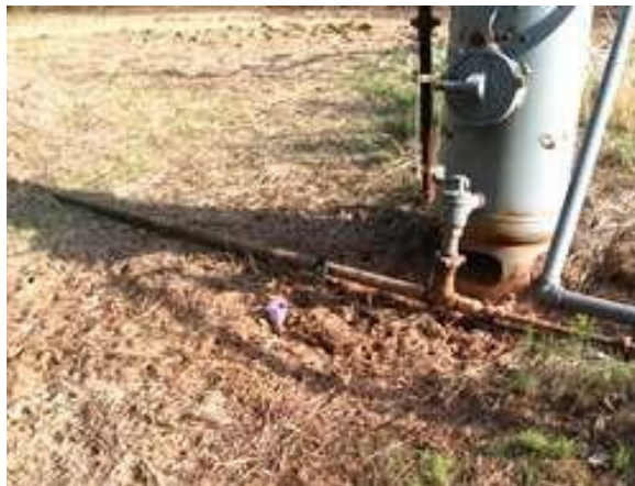
Photo 3. Pipe for oil and brine running from separator to tank (not shown). Great numbers of deer tracks along here to right up against separator.
